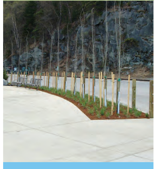
Figure 16. Urban stormwater collection used with a vegetated edge.
