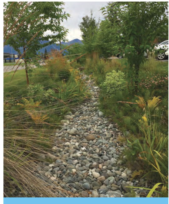
Figure 14. Bioretention swale in the Mat-Su, used to infiltrate and treat stormwater runoff from the surrounding residential area.
