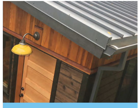
Figure 24. As an alternative to asphalt roofing material containing polycyclic aromatic hydrocarbons (PAH's), standing seam metal roofs are fire resistant, long lasting, 100% recyclable and, because they protect water quality, can be used for rainwater harvesting. Source: Salmon-Safe
