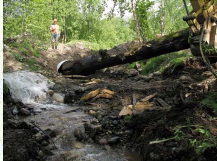
Incorrect Woody Debris Placement.
